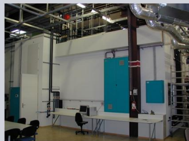
Test room Siemens HVAC Laboratory
